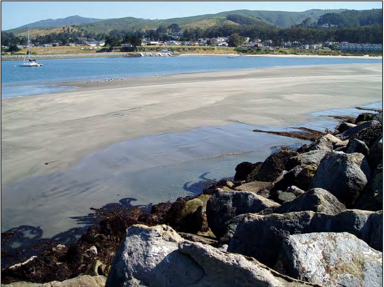
Figure 48. Photograph looking into Pillar Point Harbor showing surging of water through the east breakwater (Source: Craig Conner)
